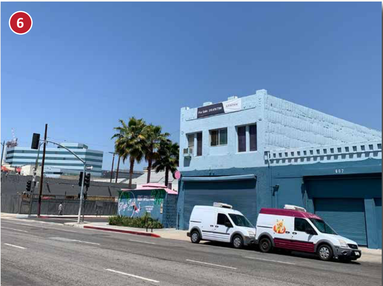
E 4th St , across street facing subject site. Direction: North
