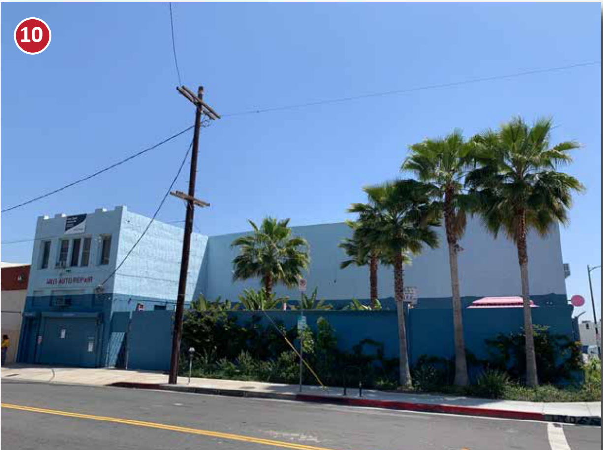
Towne Ave , across street facing subject site. Direction: East
